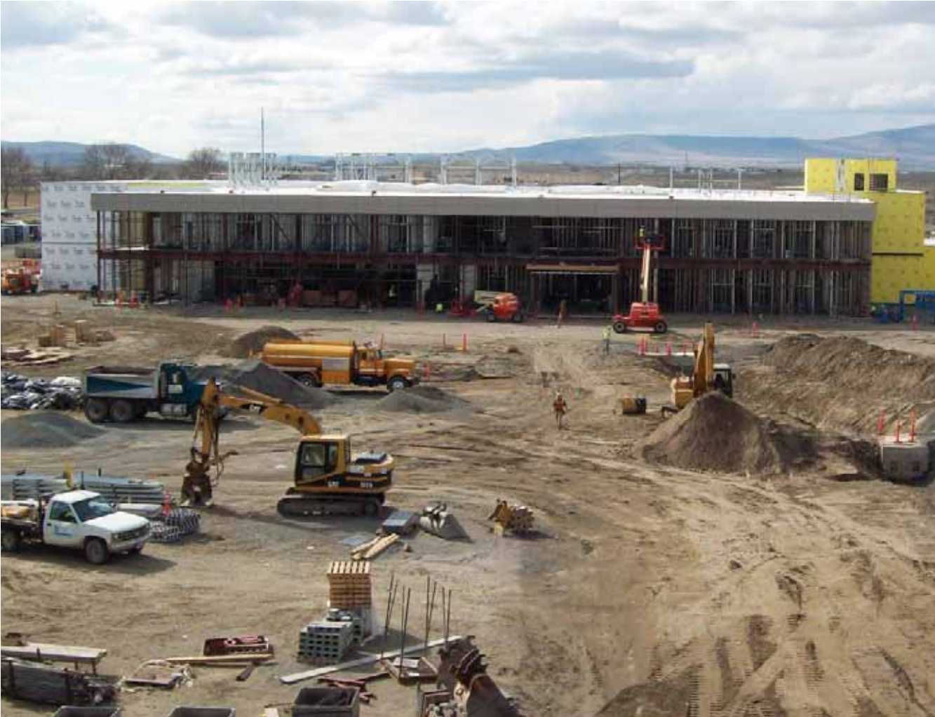
(IMAGE COURTESY OF LYDIG CONSTRUCTION CO.)
