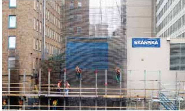
(IMAGE COURTESY OF SKANSKA BUILDING USA)
