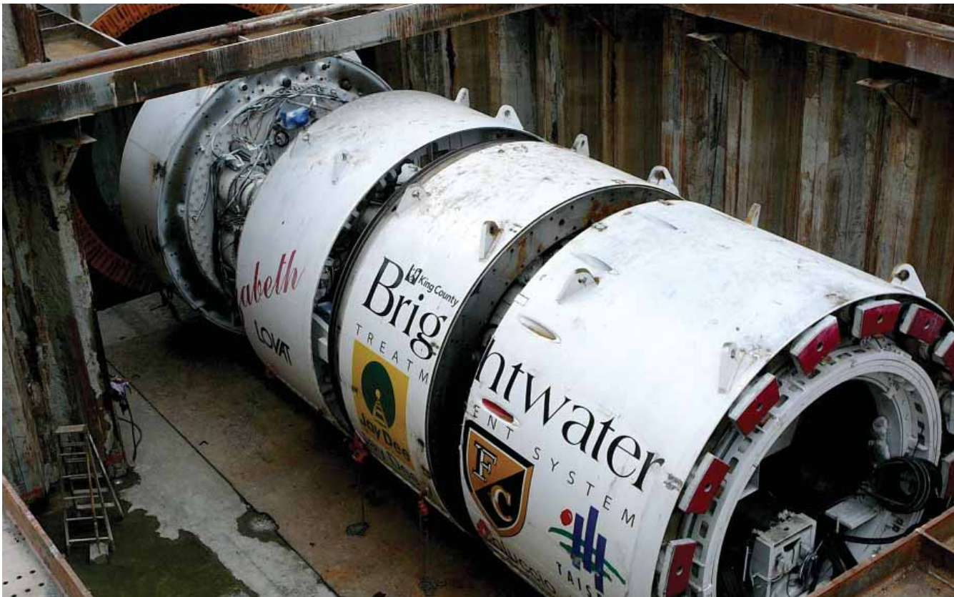
(IMAGE COURTESY OF WEST TUNNEL TBM)
